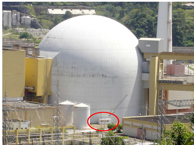
Fig. 1. Photo of the neutrino laboratory just outside the Angra II reactor containment building.
